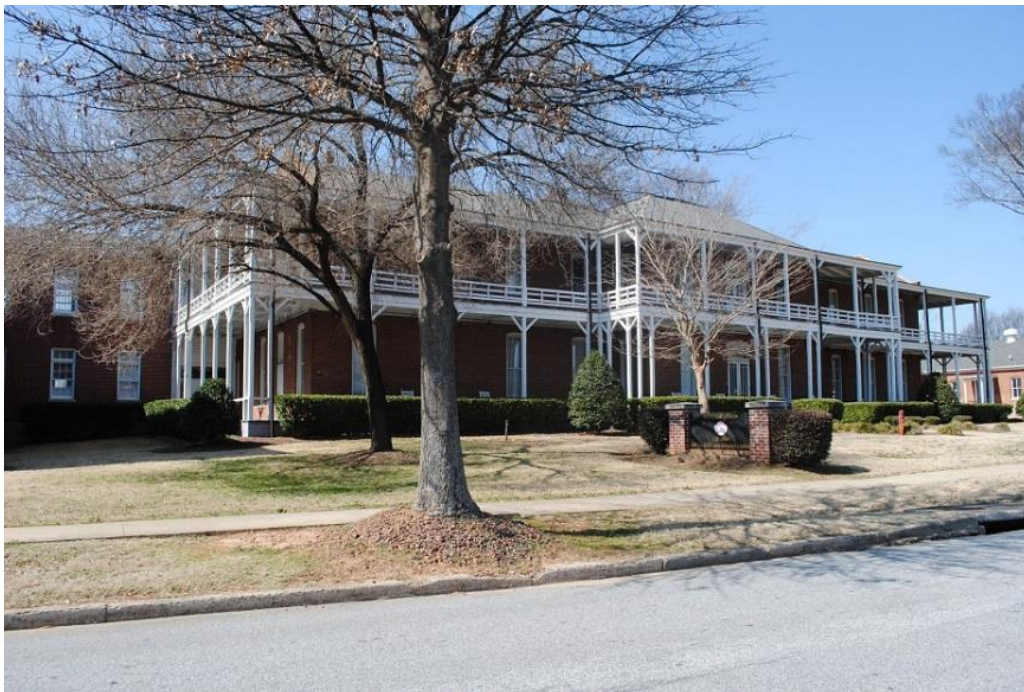
Building 171: Front façade
