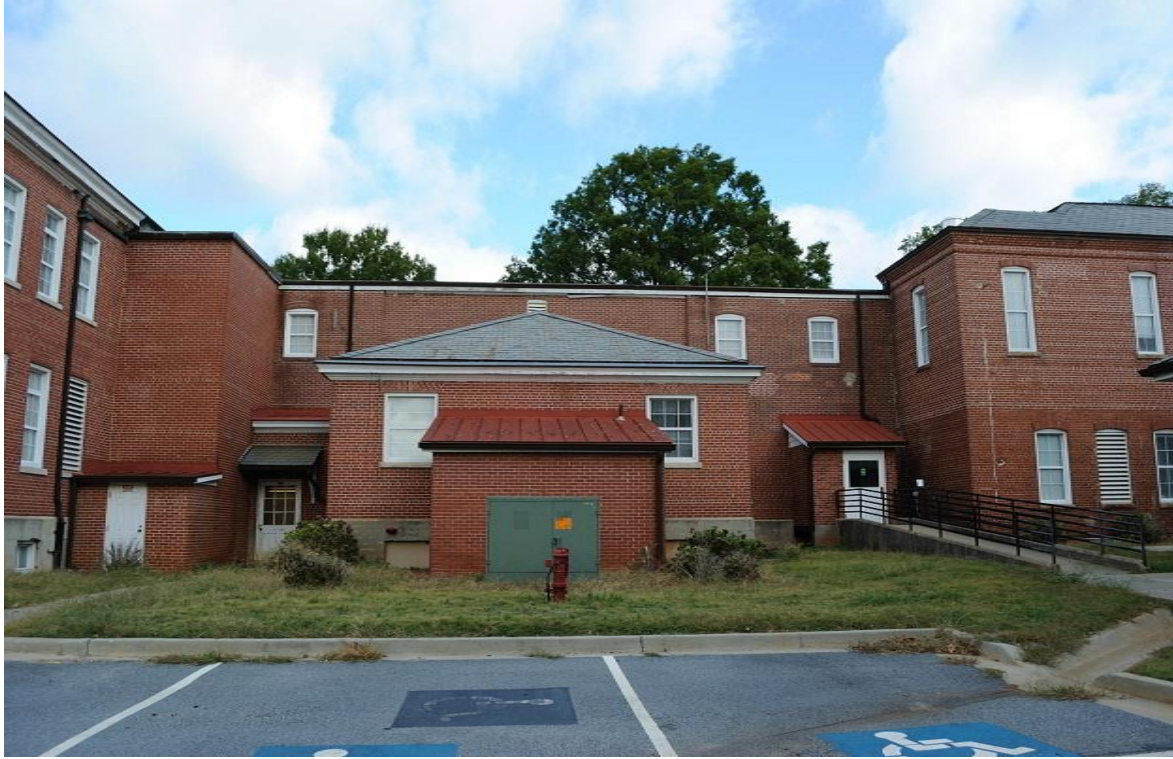
Building 171: Side (south-central section) elevation
