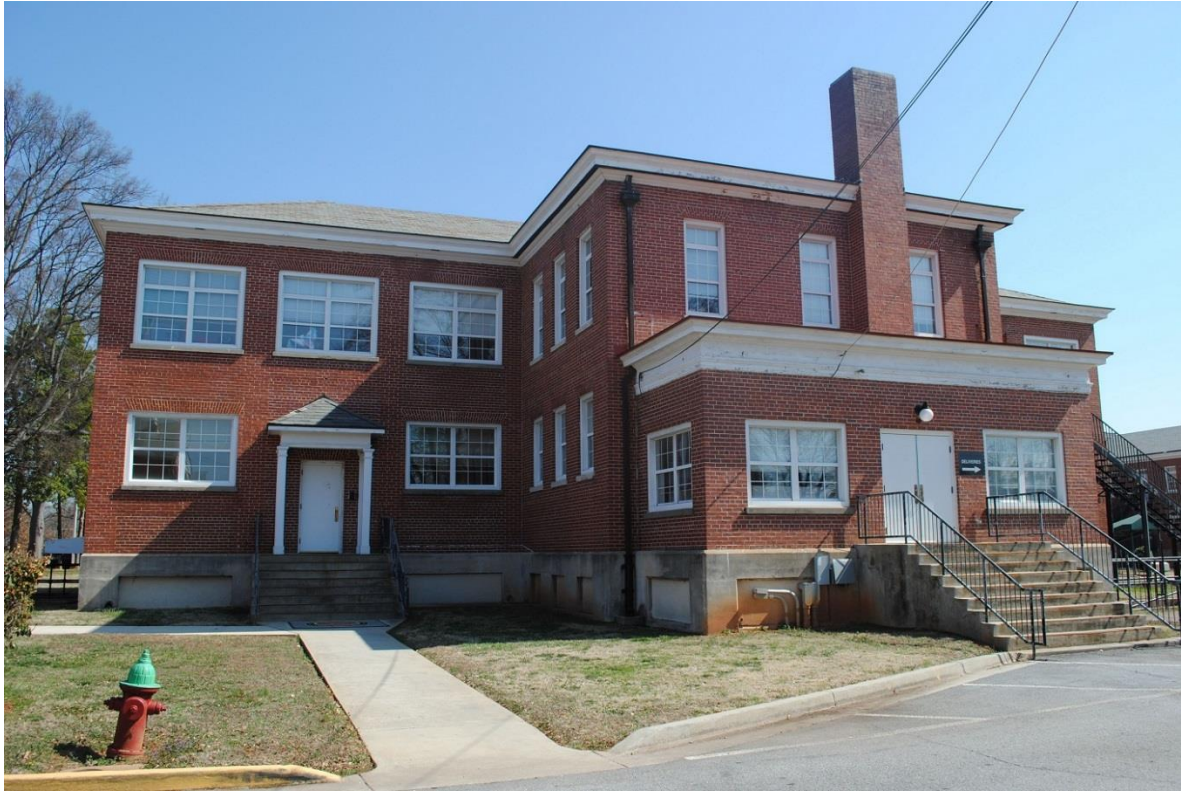
Building 171: North end of rear (west) elevation
