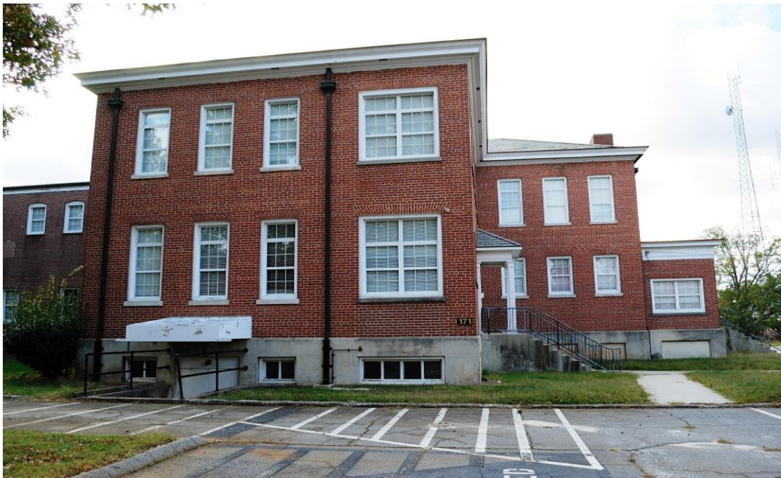
Building 171: Side (north-western section) elevation
