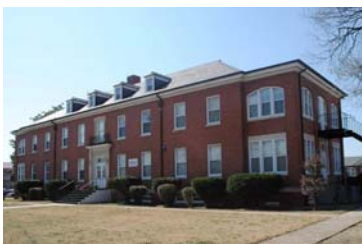
Building 168, built in 1933 was used as nurses' and transient quarters.
