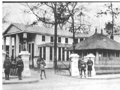
The Red Cross building (Building 46) is another architectural asset, whose fate should be carefully considered as an integral part of the Historic Village development strategy. This may be a long-term option for housing a museum.
