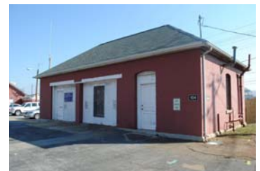
Building 104, built in 1897 was used for administrative purposes.
