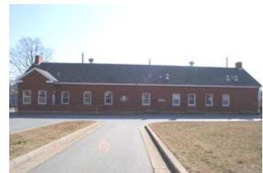
Building 100, built in 1897 was used for administrative purposes.
