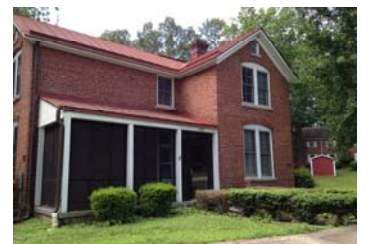
Building 532, built in 1887 served as a family headquarters.
